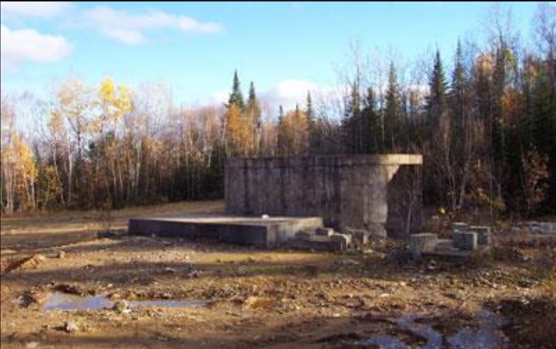
Anacon Shaft Entrance
