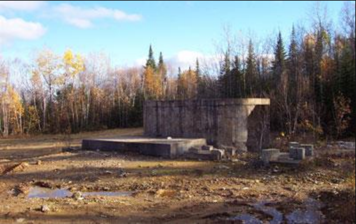
Anacon Shaft Entrance
