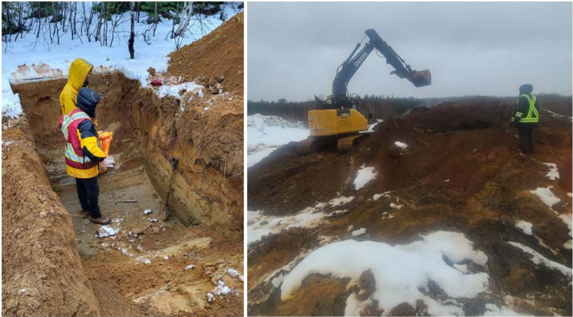
Figure 9.3: Typical test pit excavations
