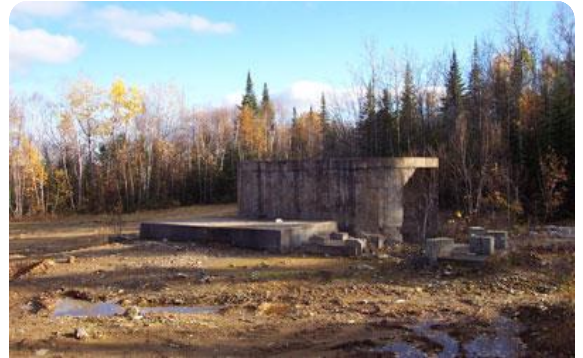
Anacon Shaft Entrance
