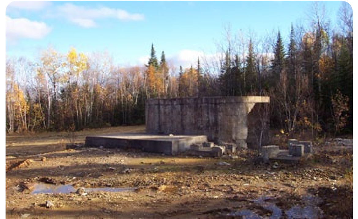
Anacon Shaft Entrance
