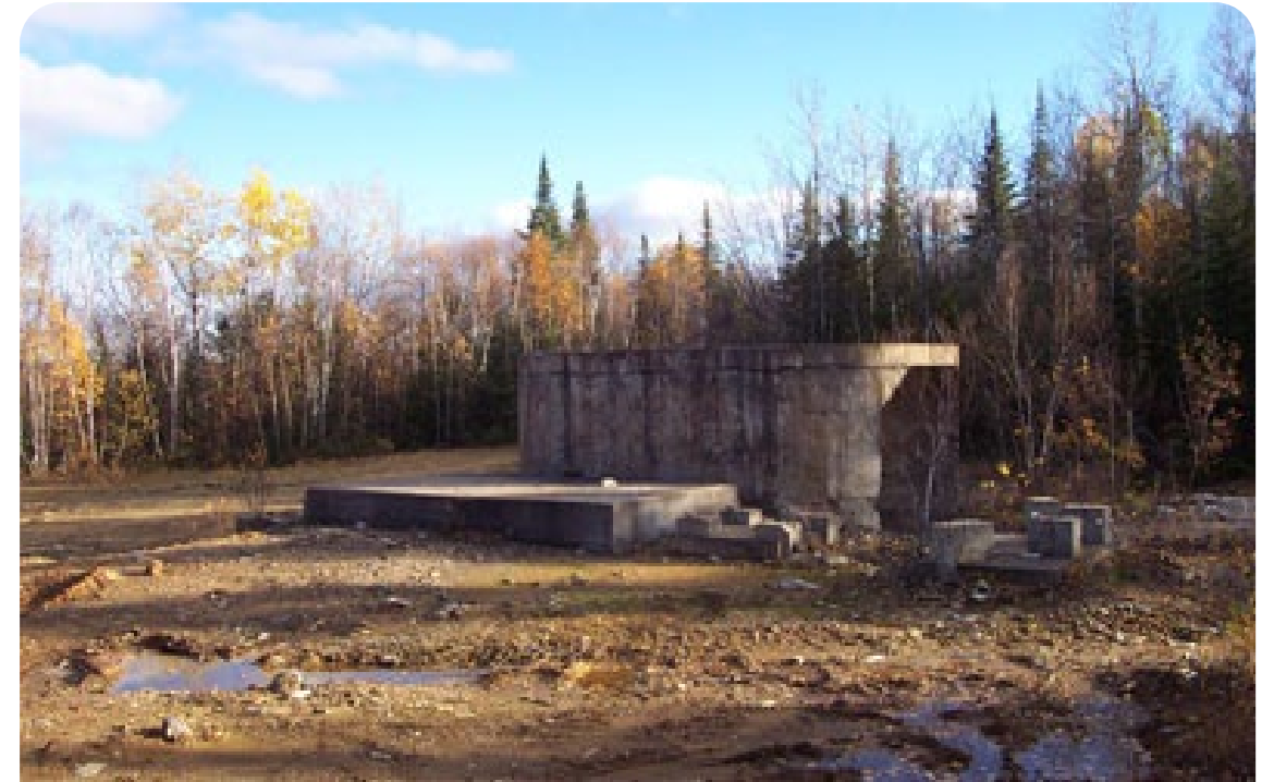
Anacon Shaft Entrance
